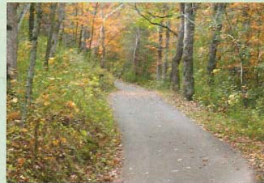
Winding up the grade. By traversing up a steeper grade with modest switchbacks and landings, this trail is less imposing (and more fun) than it might otherwise be if the trail climb were more direct.
