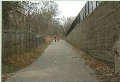
Ramp up to old rail grade. Although this ramp exceeds 5 percent, it is short enough for most people to negotiate. This could have been improved by providing larger landing areas at top and bottom.
