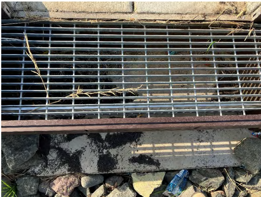
Photo 2: Stormwater Treatment Structure with minimal sediment deposition
