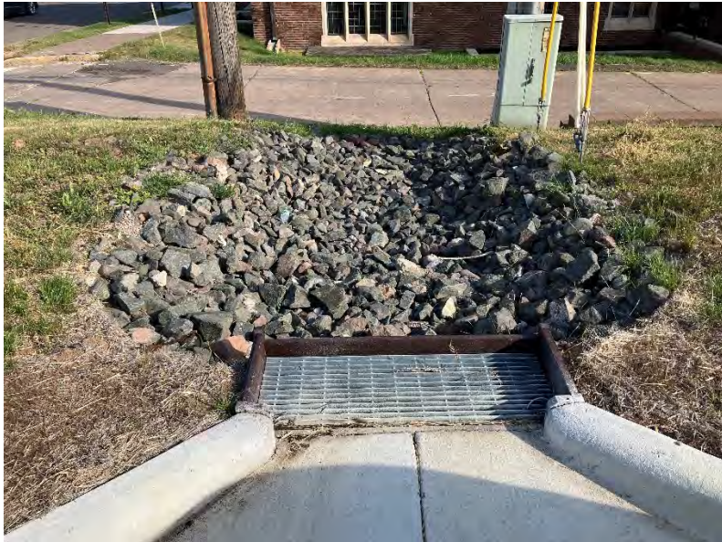
Photo 1: Stormwater Treatment Structure and Outlet showing stable conditions.
