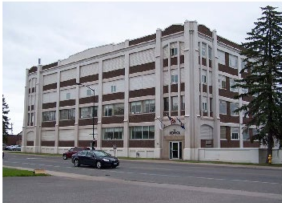
Example of Main Street Building III
