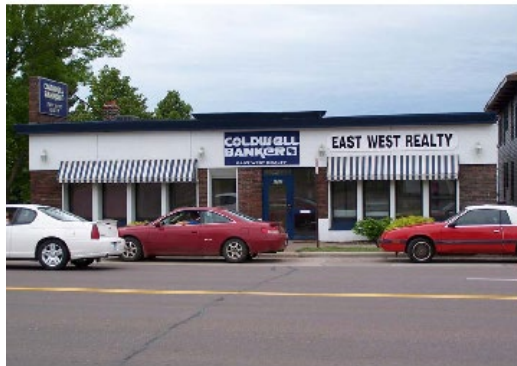
Example of Corridor Building I
