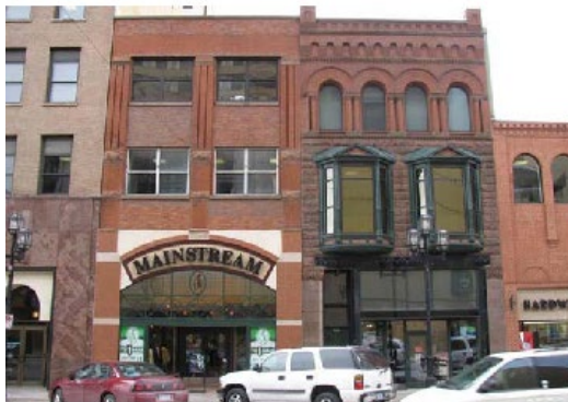
Example of Main Street Building III
