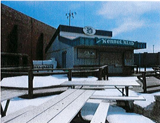
Photo 4: The 3rd base side outdoor concession stand provides a low section of counter. This is a good example of accessibility. Modify the route to the concession stand to eliminate slope and cross slope.
