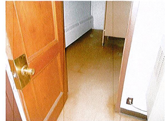
Photo 3: The entry door to the toilet room currently provides a 26 1/2" clear opening.
