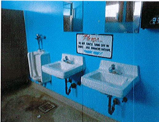
Photo 4: Insulate the pipes at the sink.
