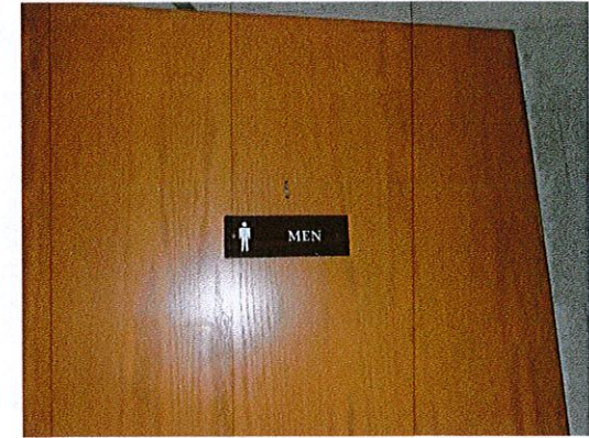
Photo 6: Add signs with raised and braille characters to the toilet rooms.
