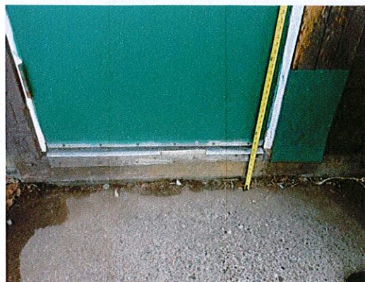
Photo 2: Patch the rise at the lower level entry.
