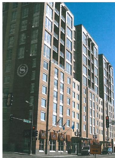
Example of Corridor Building III
